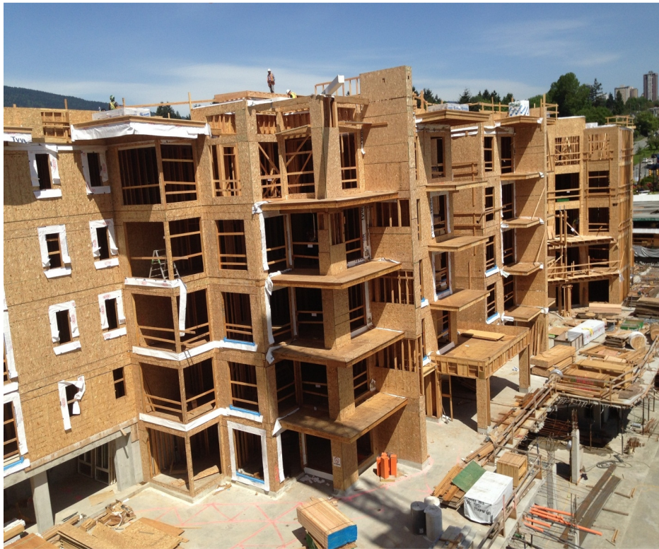
Photo of midrise wood frame building under construction. Source: Steven Street, Ontario Wood Works!
